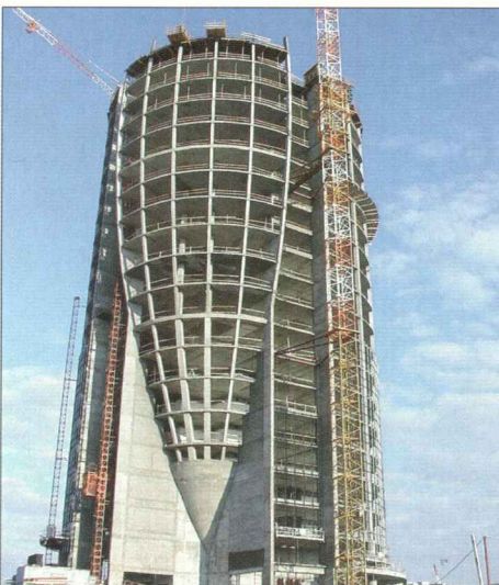
Fig. 6: Eastern spatial wing at construction
